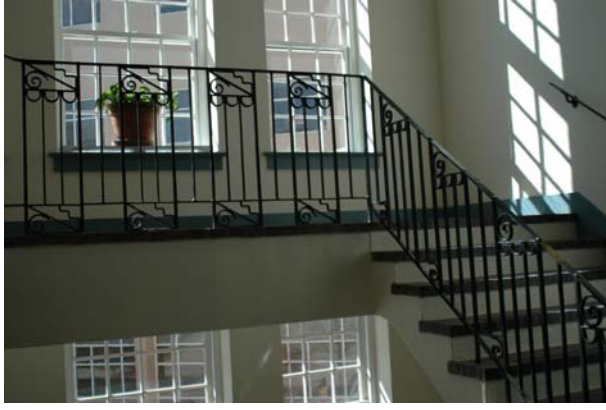
The distinguishing features of the historic Villagra Building were preserved, such as its large double-hung windows, wrought iron railings, and brick stair treads.
