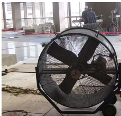
Figure 40: Photographs showing air quality management practices by the contractor during various phases of construction. From top to bottom: Ducts are sealed with plastic immediately after installation to prevent entrance of dust, dirt, or water (SMACNA 3.2 HVAC protection); protect materials from exposure to moisture (SMACNA 3.5 Housekeeping); a fan provides additional ventilation during painting and finishing operations (SMACNA 3.3 Source Control).
