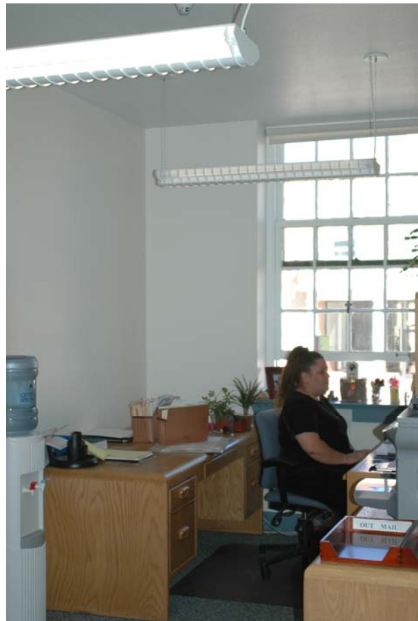
Offices in the Villagra Building feature operable windows for daylight and ventilation. Daylighting sensors illuminate the lights farthest from the window, while the lights closest to the window are automatically turned off or dimmed to save energy.
