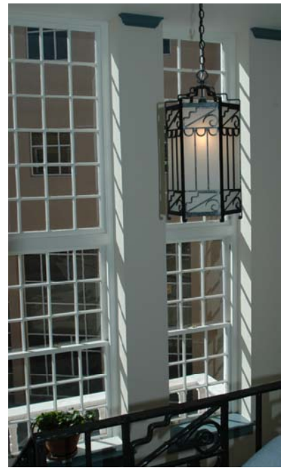
Thermal properties of the original windows were improved by applying a high-tech ceramic film called Huper Sech to the interior glass surface.
