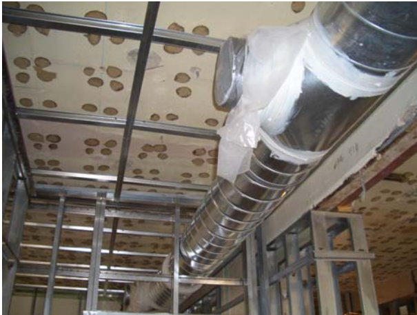
Ceiling ducts were protected with plastic from dust and moisture during construction.
