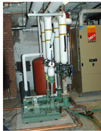
New compact boiler plant.
