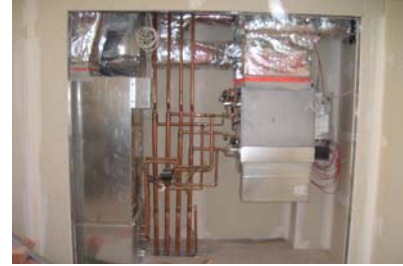
HVAC units fit compactly into office closets as a result of creative problem-solving by the mechanical contractor and team. Fan coil units consist of a fan, heating and cooling coil, and filter.
