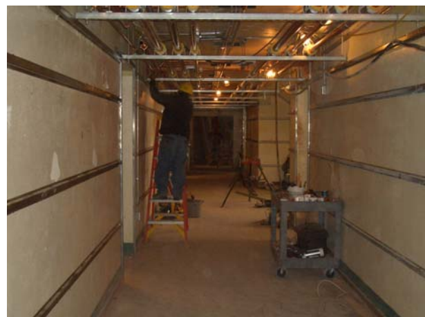
New four-pipe HVAC installation in the basement ceiling.
