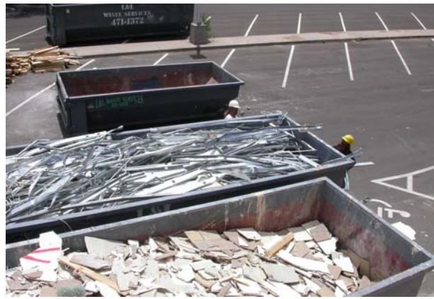
Roll-offs in the parking lot of the building enabled construction crews to separate waste for reuse and recycling, contributing to an overall construction waste reduction of 82%.
