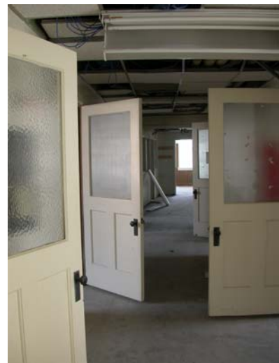
The building's original doors were reused.
