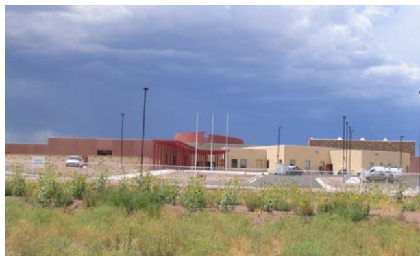
Figure 10: The Baca Dlo'ay azhi Community School, located in Prewitt, New Mexico, was the first building in the state to receive LEED certification. The building earned a rating of LEED Certified in January 2004.
